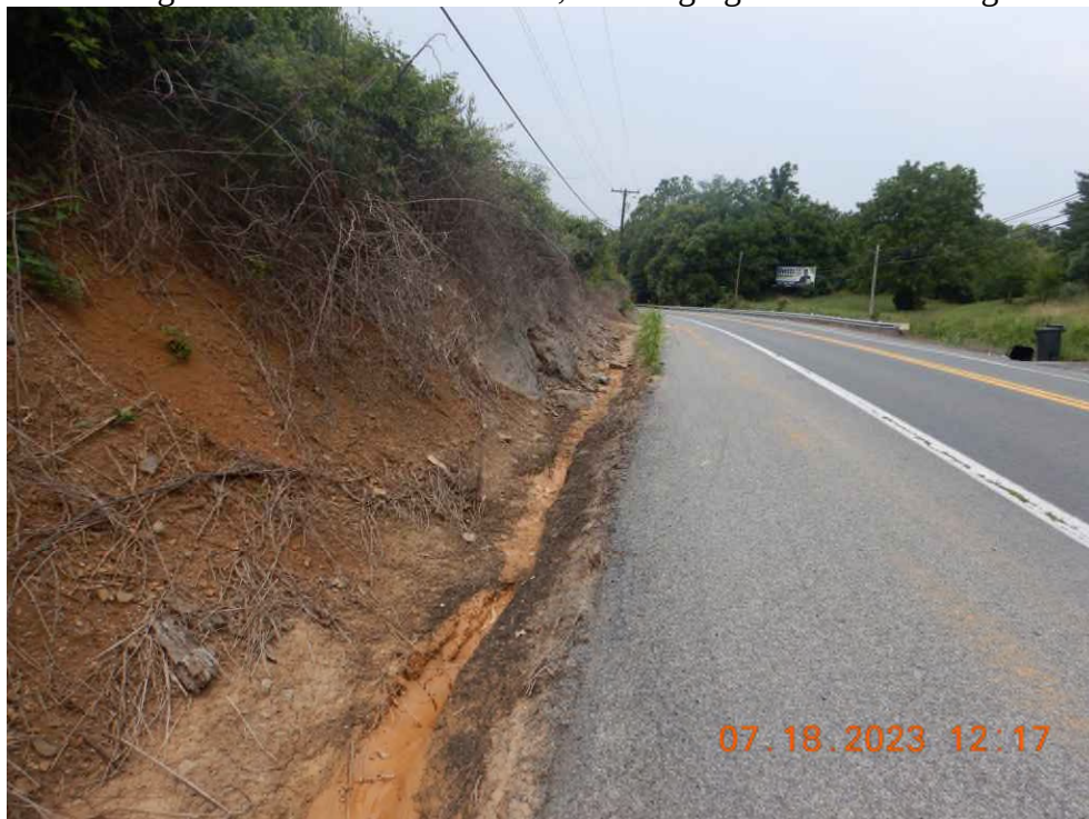
Sediment laden water leaving the project area through WVDOH right of way.
