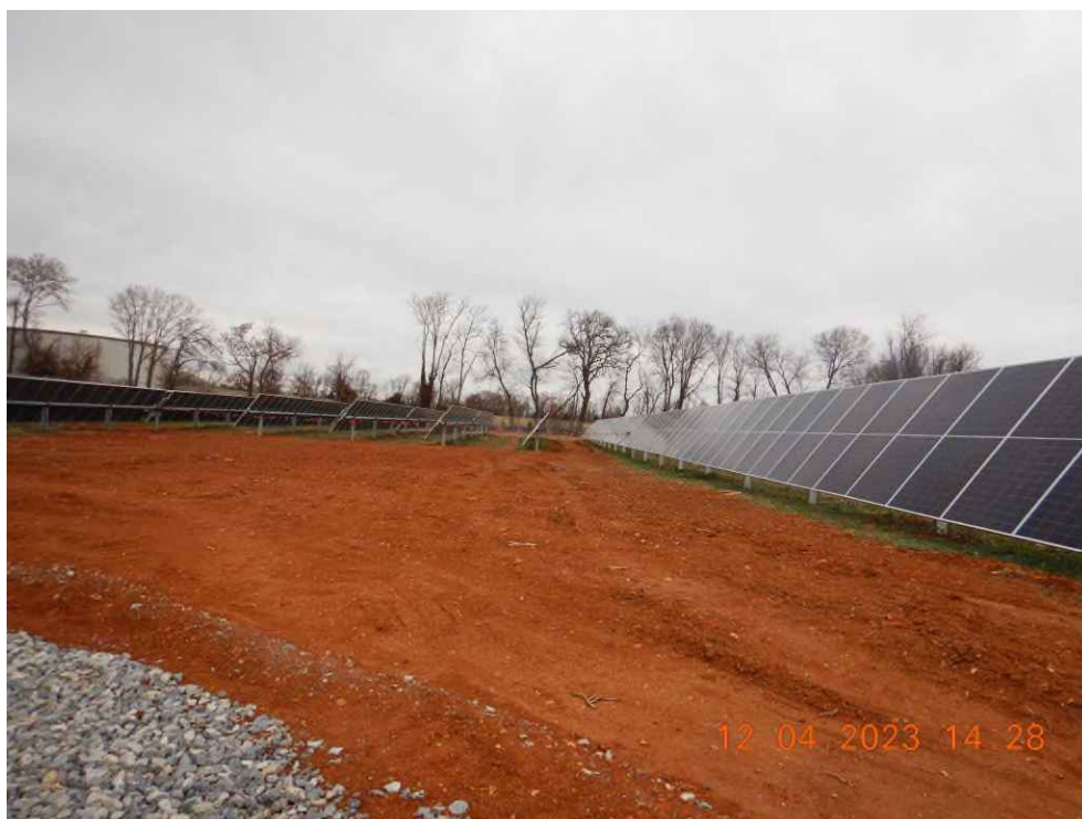
Area where Sediment Trap 5 should be installed.
