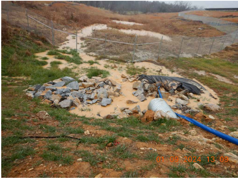
Sediment Basin 13 discharging into Evitts Run.
