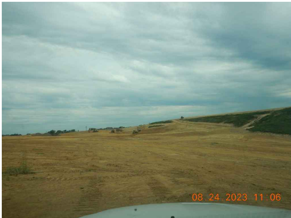
Area that lacks stabilization.
