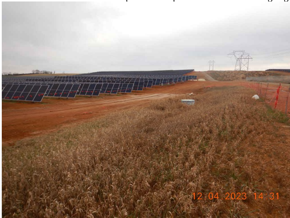
Sediment Basin 10 converted to Pond 8 prior to all upstream disturbance being vegetated.
