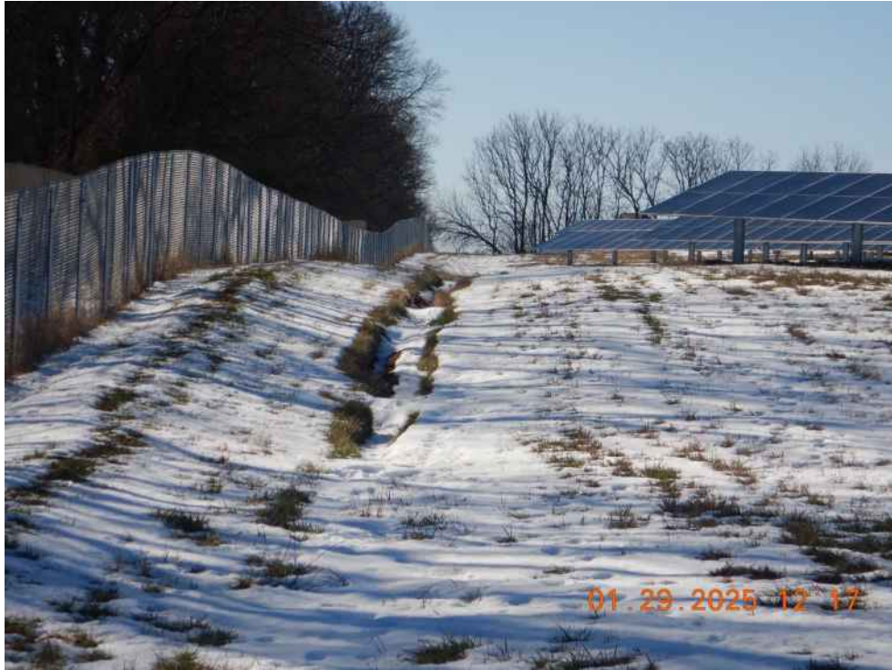
An unstabilized/washed out diversion channel.
