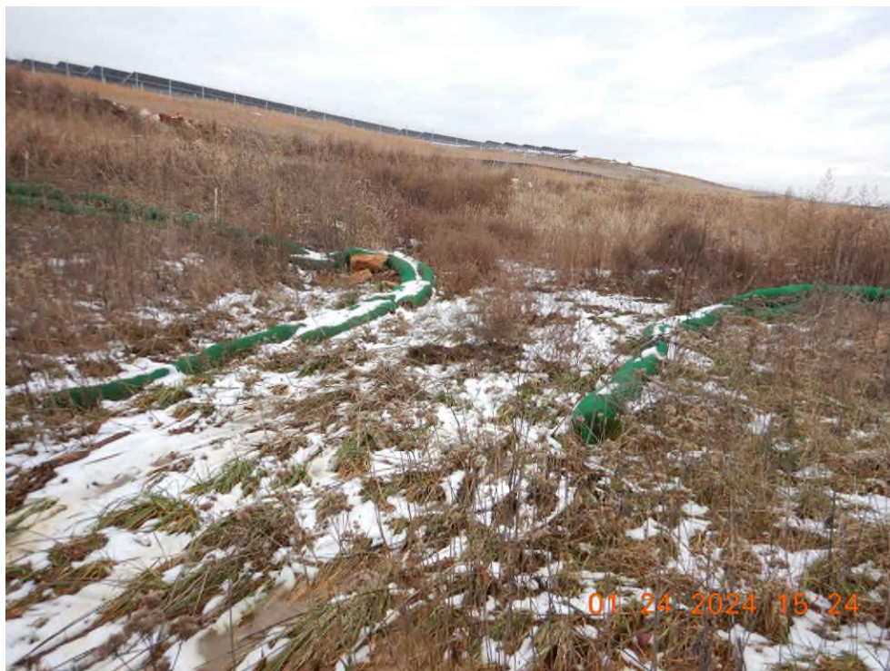
Sediment laden water leaving site downslope of Basin 13.
