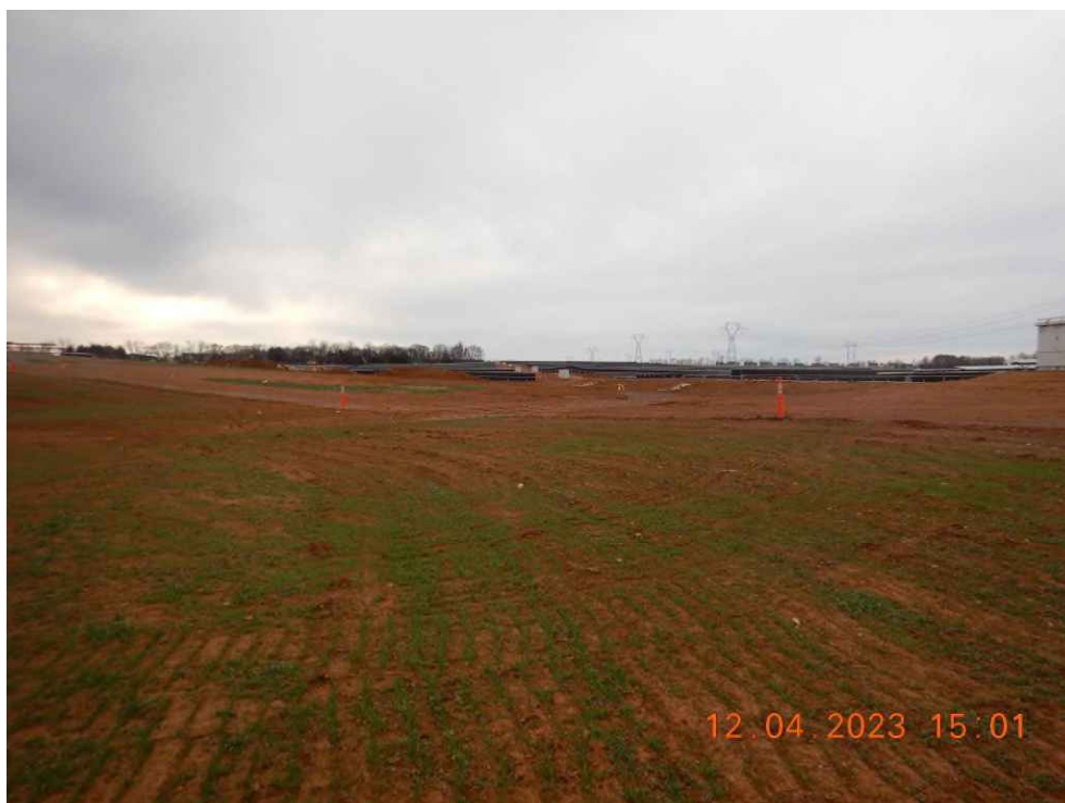
Area where sediment Basin 17 should be installed. Basin has been removed prior to all uphill disturbance being vegetated.
