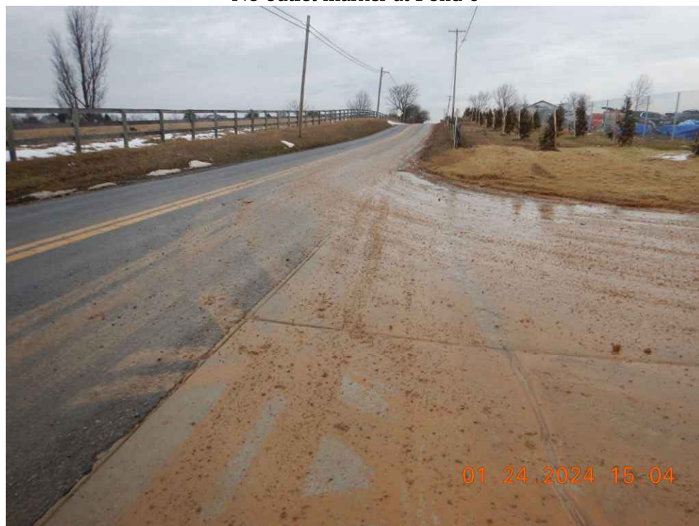
Track-out from Construction Entrance 2 that was not being cleaned during inspection.
