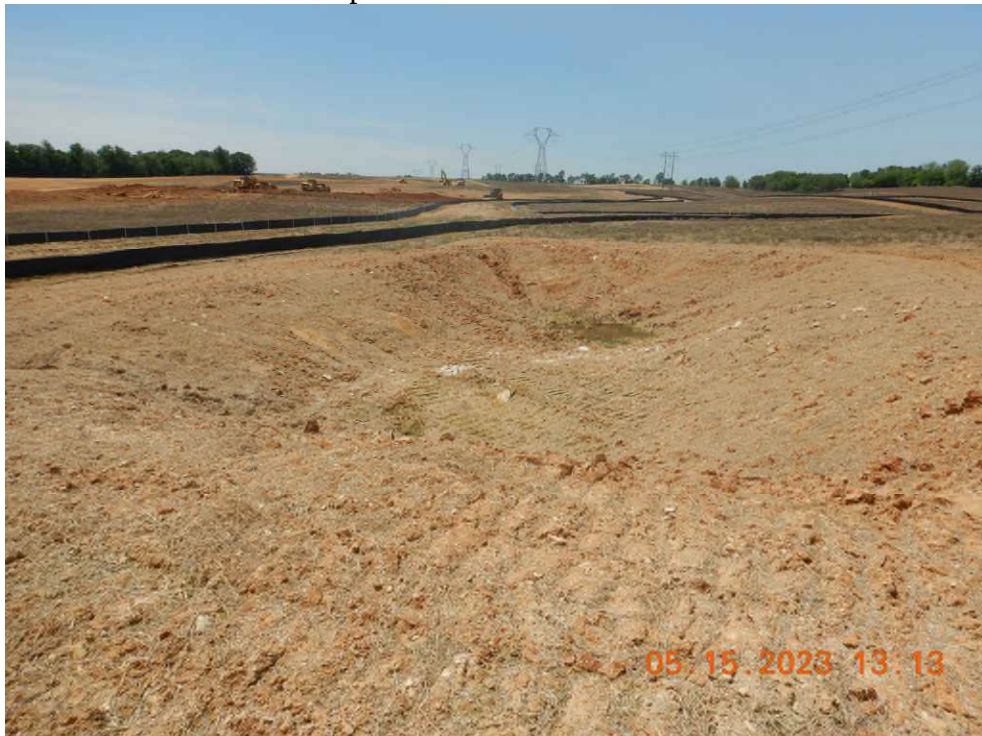
Sediment Trap 16 has no stabilized inlet or outlet.
