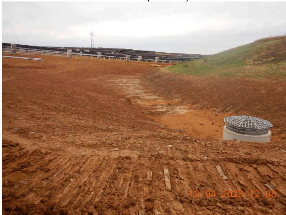
Sediment Basin 1 has been converted to Pond 3A prior to all upstream disturbance being vegetated.
