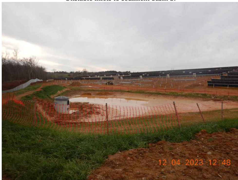
Sediment basin 3 (Pond 3B) converted prior to all uphill disturbance being vegetated.
