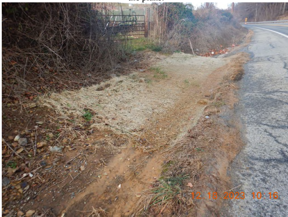
Sediment laden water leaving site via outlet of Sediment Basin 6.
