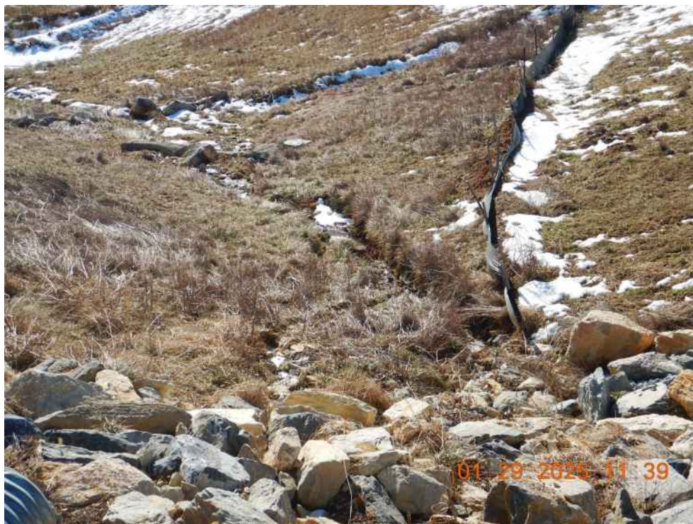
An unstabilized channel that has eroded due to lack of vegetation.
