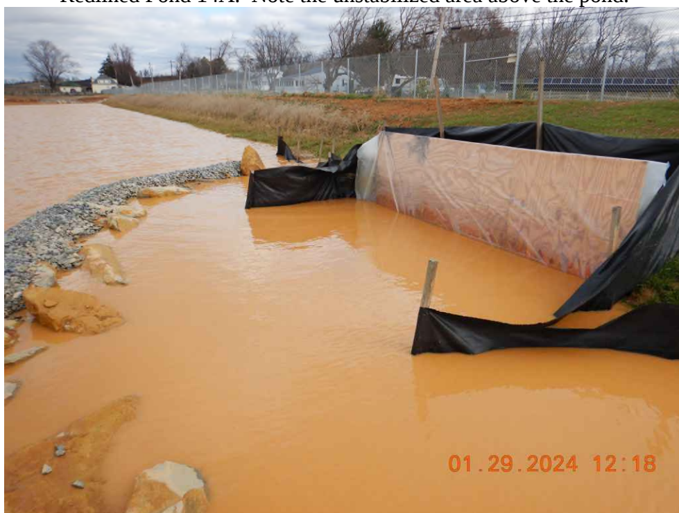
Outlet of pond 14A discharging offsite.
