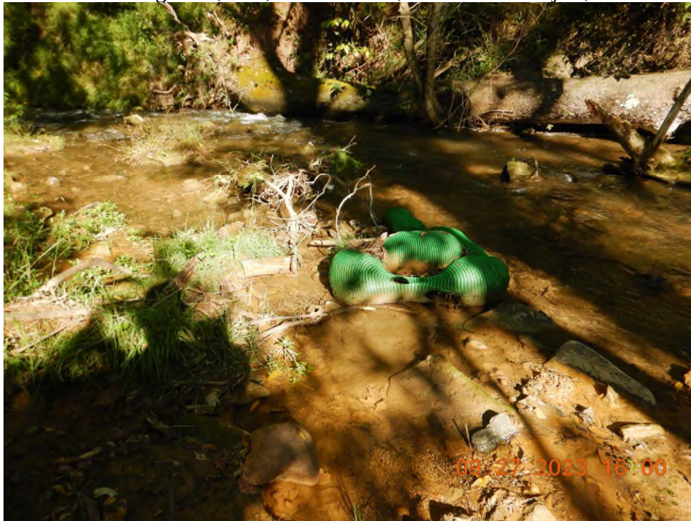
Conditions not allowable - deposits in Evitts Run (39° 15' 17.2288" X -77° 49' 26.9350") from Sediment Basin 5. Filter sock laying in creek.
