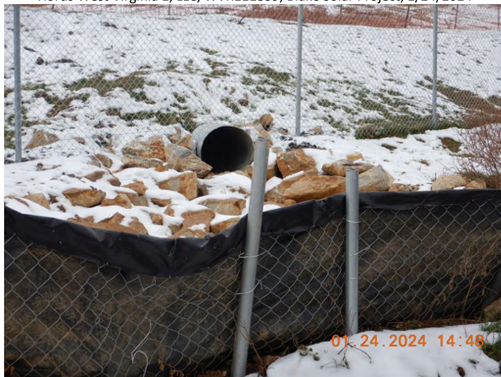
No outlet marker at Pond 6
