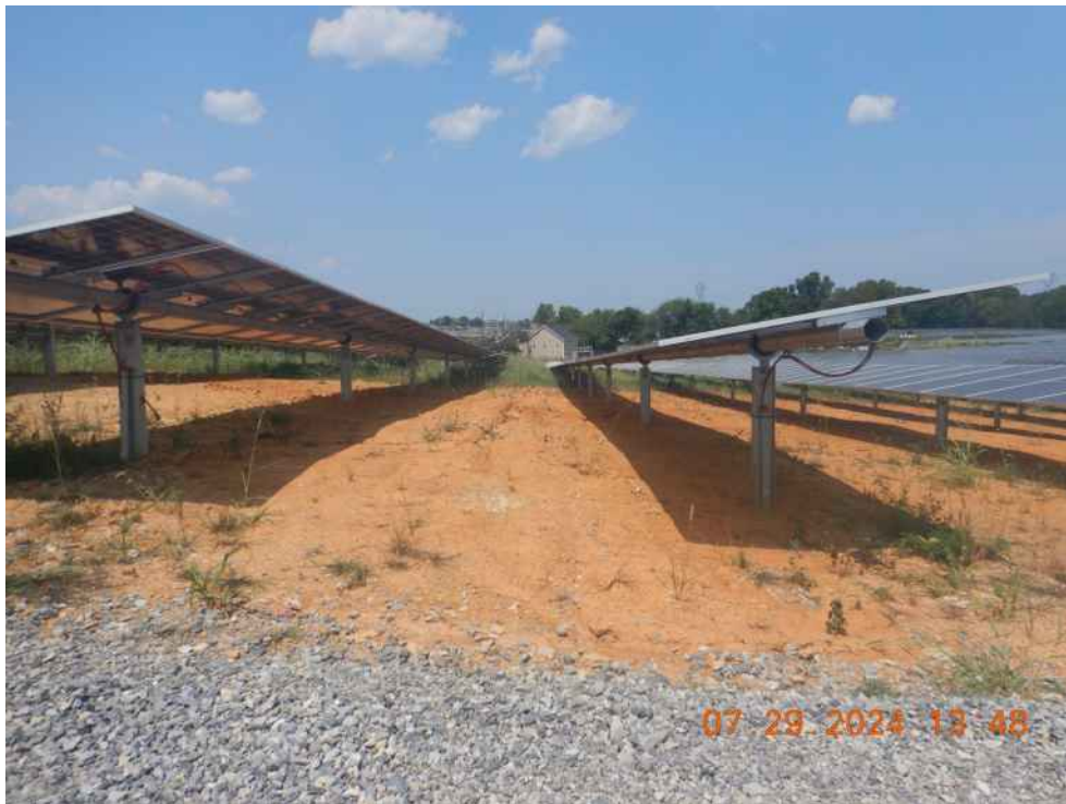
An unstabilized area that has not been actively worked. Sediment basin 17 drainage area.
