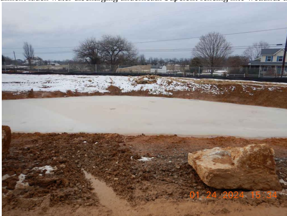
New pond that has been installed to prevent sediment laden water from leaving the site. SWPPP needs to be modified to include pond.
