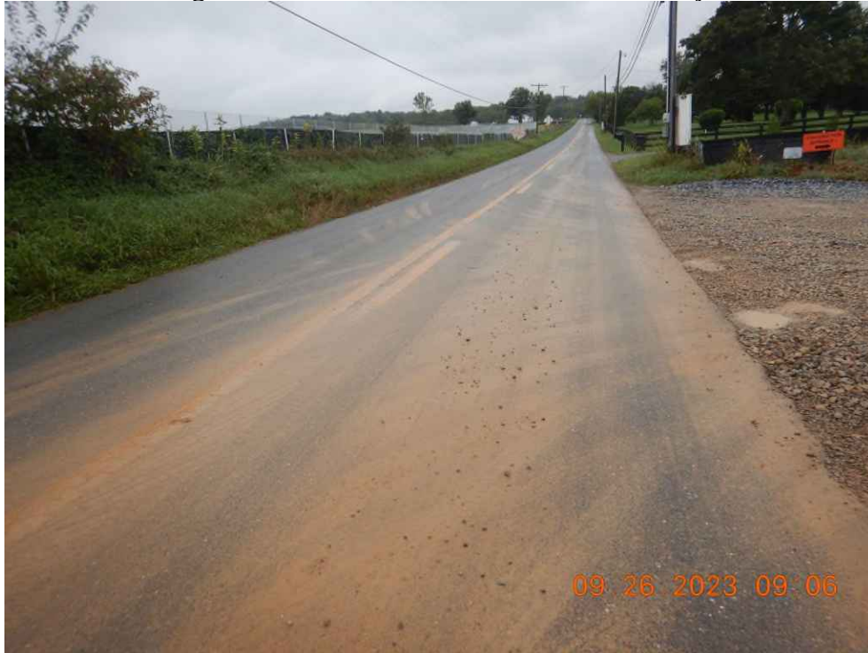
Track-out from the site on Kabletown Road.
