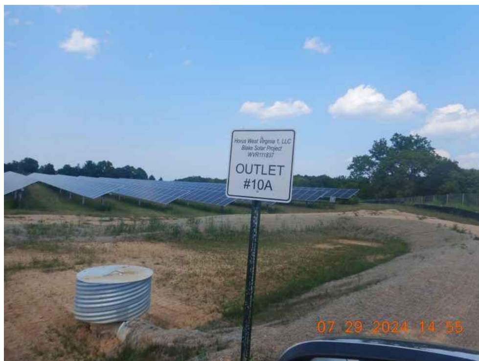
Sediment basin 9, that has been converted prior to all uphill disturbance being stabilized.
