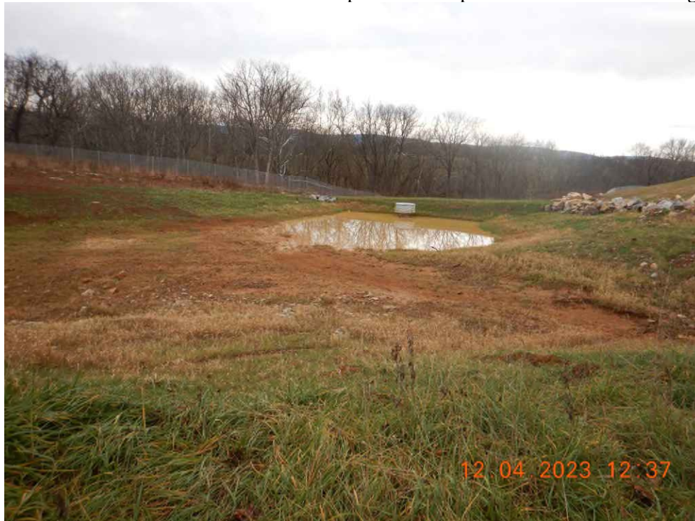
Sediment Basin 6 has been converted to Pond 4B prior to all upstream disturbance being vegetated.
