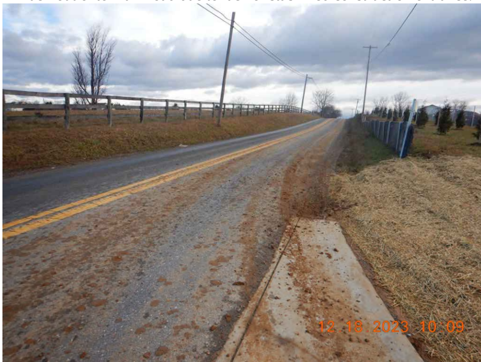
Track-out onto main road due to lack of stabilized construction entrance.
