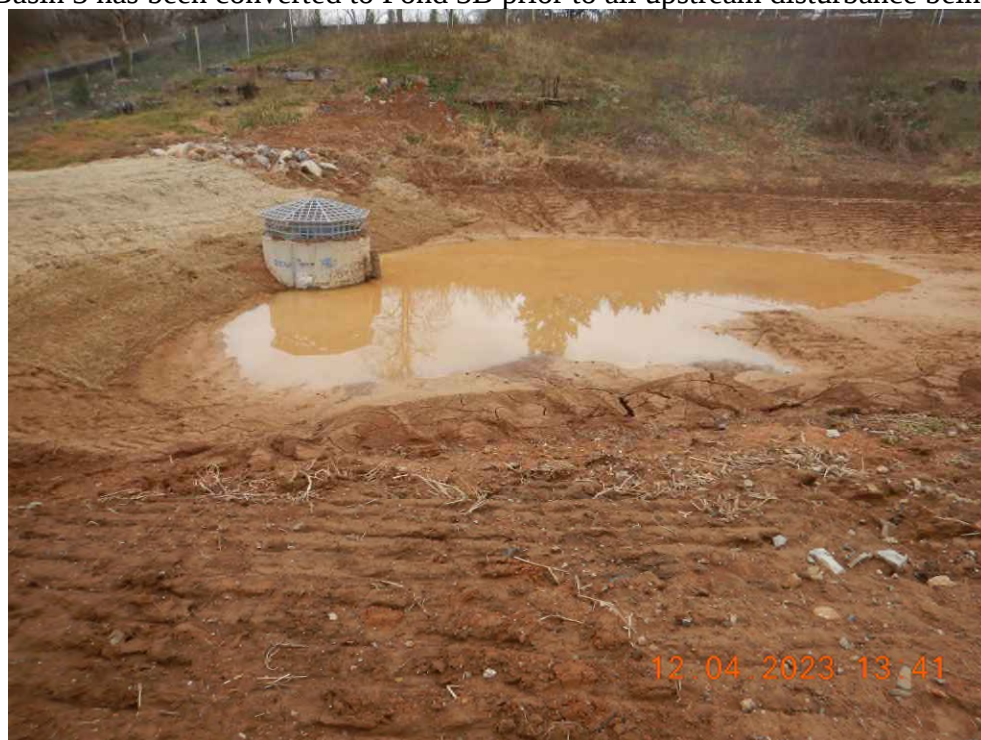
Sediment Basin 15 has been converted to Pond 1 prior to all upstream disturbance being vegetated.
