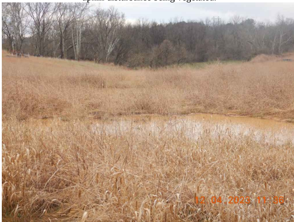
Sediment laden discharge from Sediment Basin 13 into Evitts Run.
