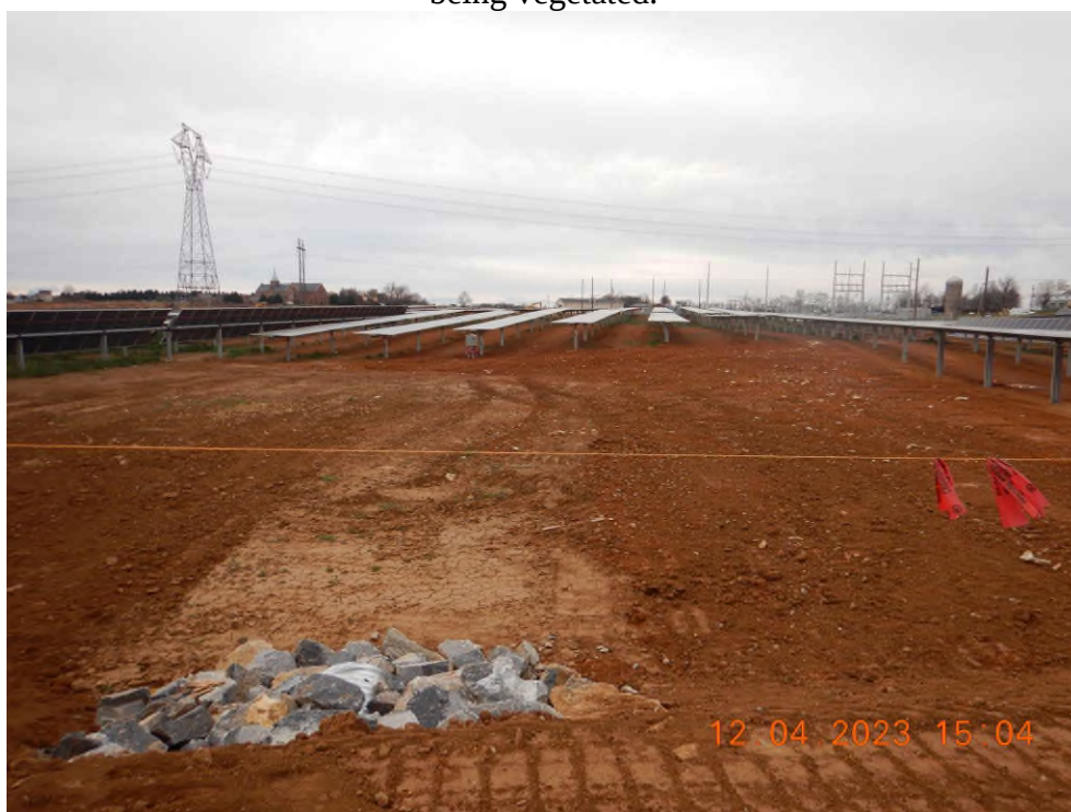
Unstabilized area above Pond 14A.
