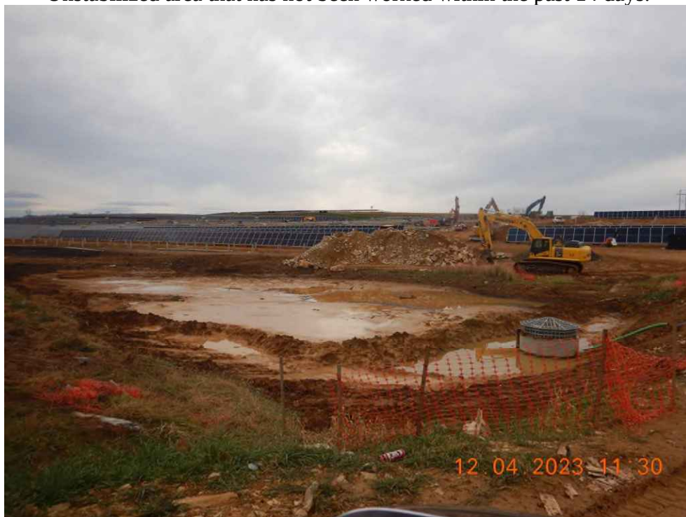
Sediment Basin 13 that has not been stabilized with outlet structure installed. Now known as Pond 2A on redline plan.
