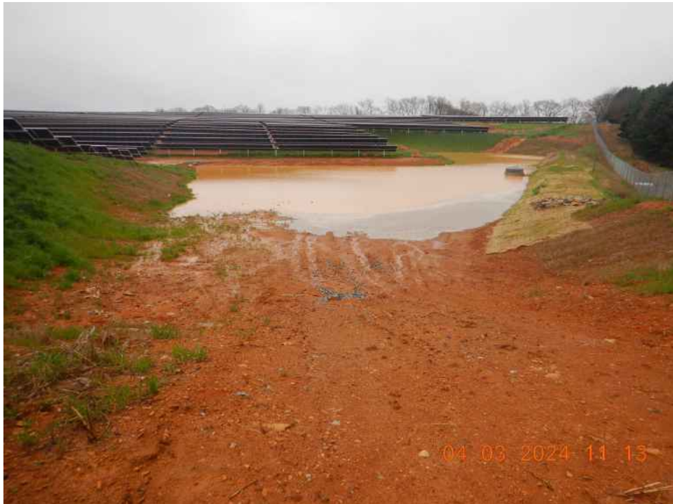
Area that has not been worked in the past 14 days and lacks stabilization above Pond 16B.
