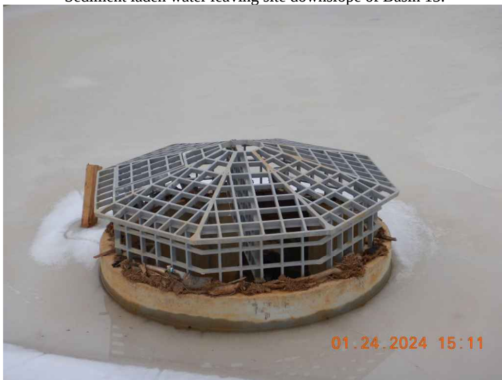
Riser for Basin 13 installed for the final stormwater pond.
