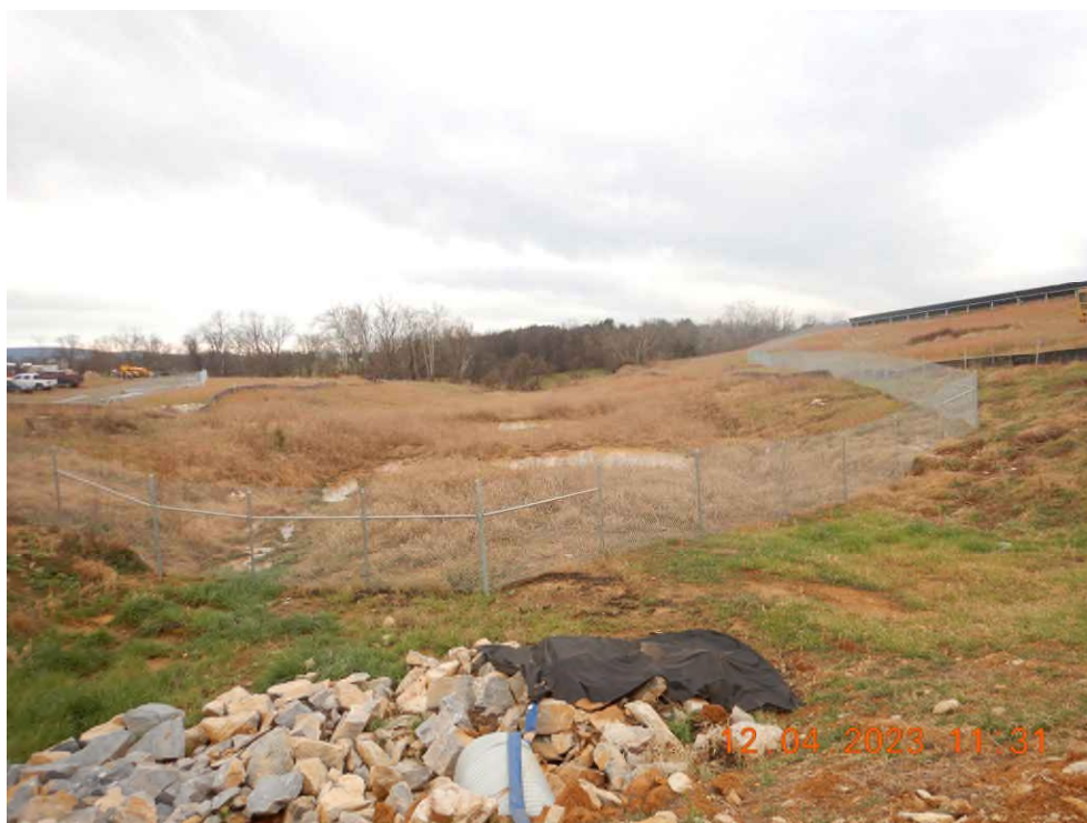
Sediment laden water leaving area Sediment Basin 13. Outlet structure has been installed prior to all uphill disturbance being vegetated.
