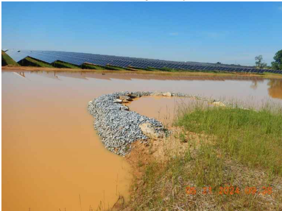
Sediment Basin 11 discharging offsite.
