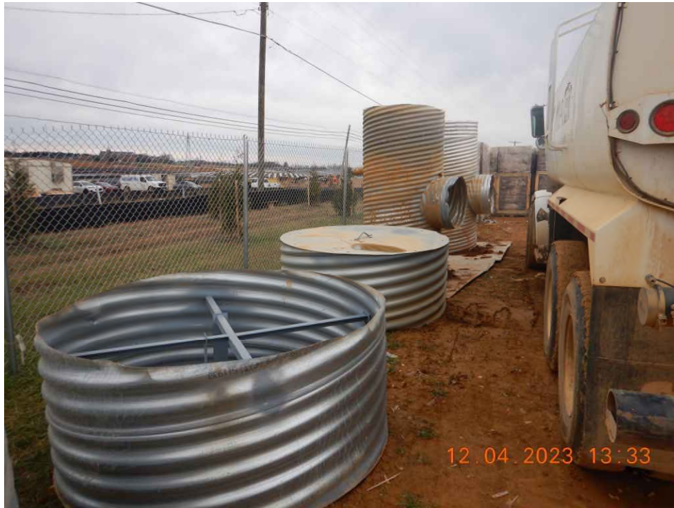
Sediment basin structures that have been removed prior to all uphill disturbance being vegetated. Stockpiled riser structures from removed trapping structures pictured.
