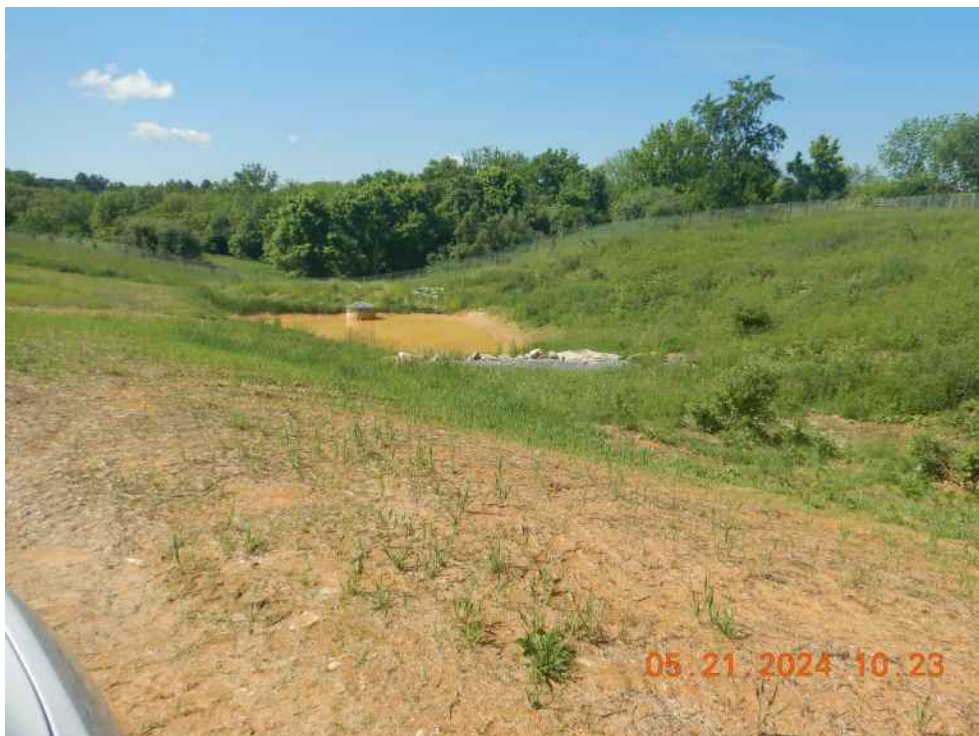
Unstabilized area above Sediment Basin 14.
