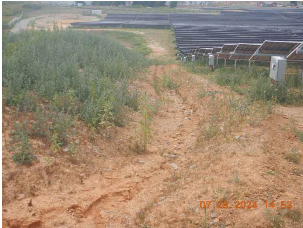
An unstabilized diversion that has not been repaired. Above sediment trap 2.
