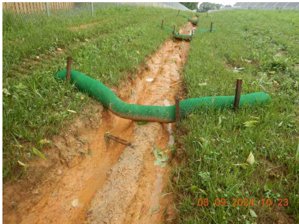
Ditch checks lack maintenance and have been undermined.
