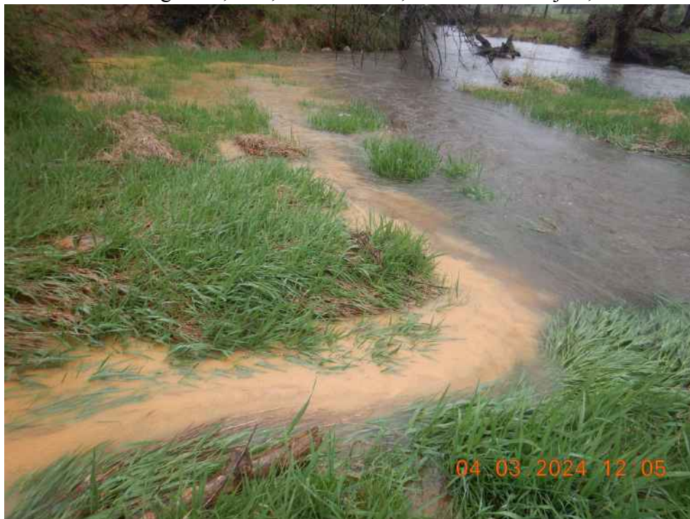
Outlet 2A discharging off site directly into Evitts Run. Causing Conditions not allowable.
