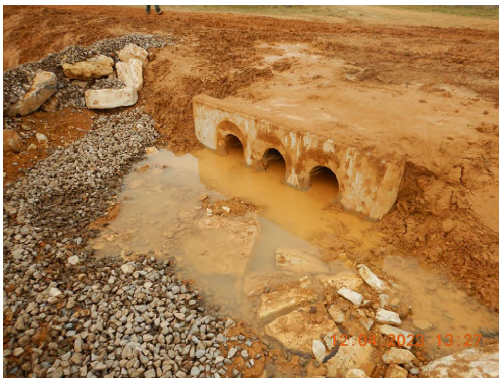
Sediment basin SB-11 (Pond 2B redline) that has been converted to stormwater retention prior to stabilization of the contributing area. Outlet pictured.
