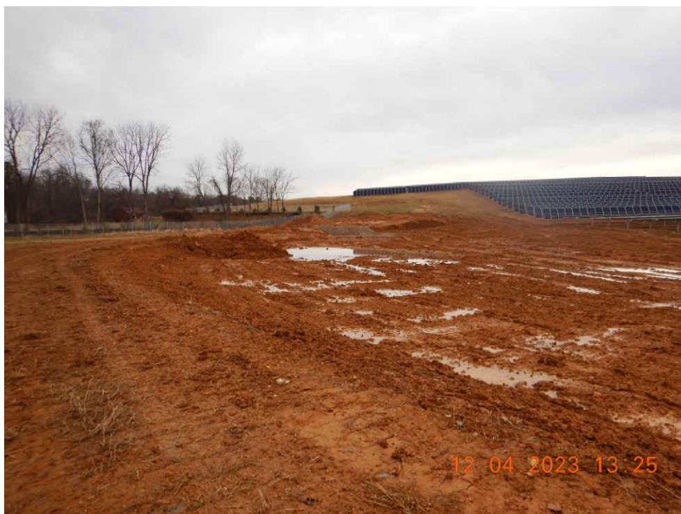
Sediment basin SB-11 (Pond 2B redline) that has been converted to stormwater retention prior to stabilization of the contributing area.
