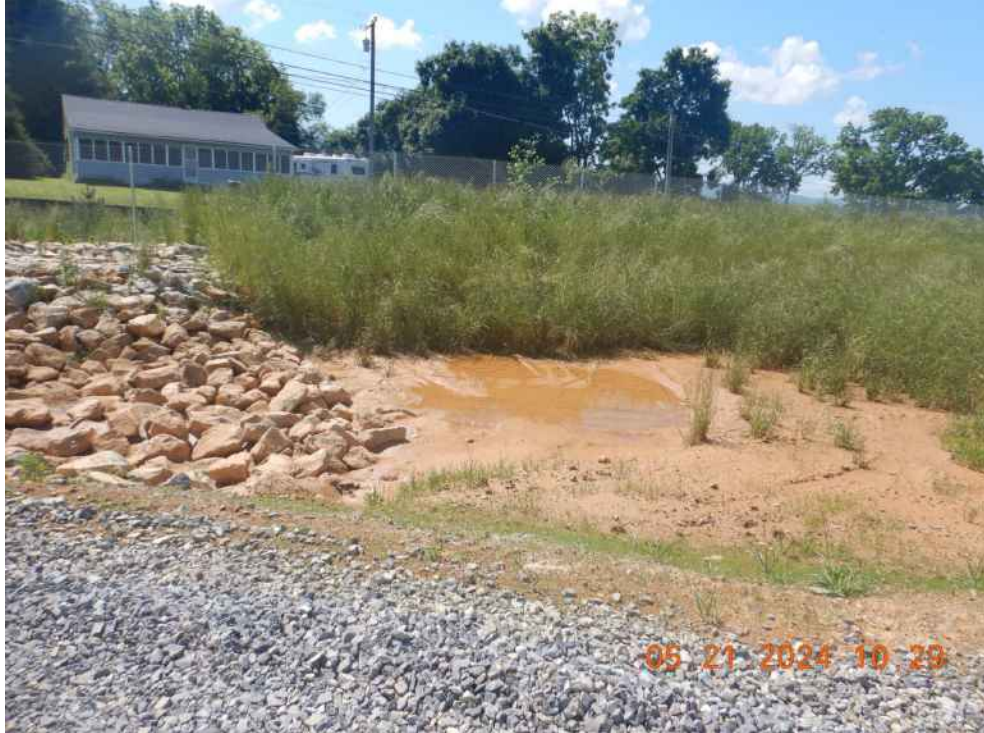
Unstabilized area above Pond 14A.
