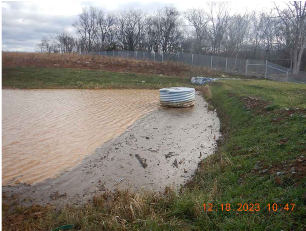
Sediment Basin 5 has been converted to final stormwater management Pond 4B. Discharging sediment laden water into Evitts Run.
