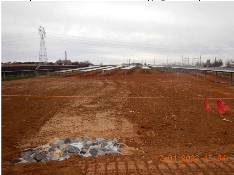
Area that has not been worked within the past 14 days and has not been stabilized. Area of proposed Sediment Trap ST-10 pictured, showing it as not in place with a disturbed contributing area.
