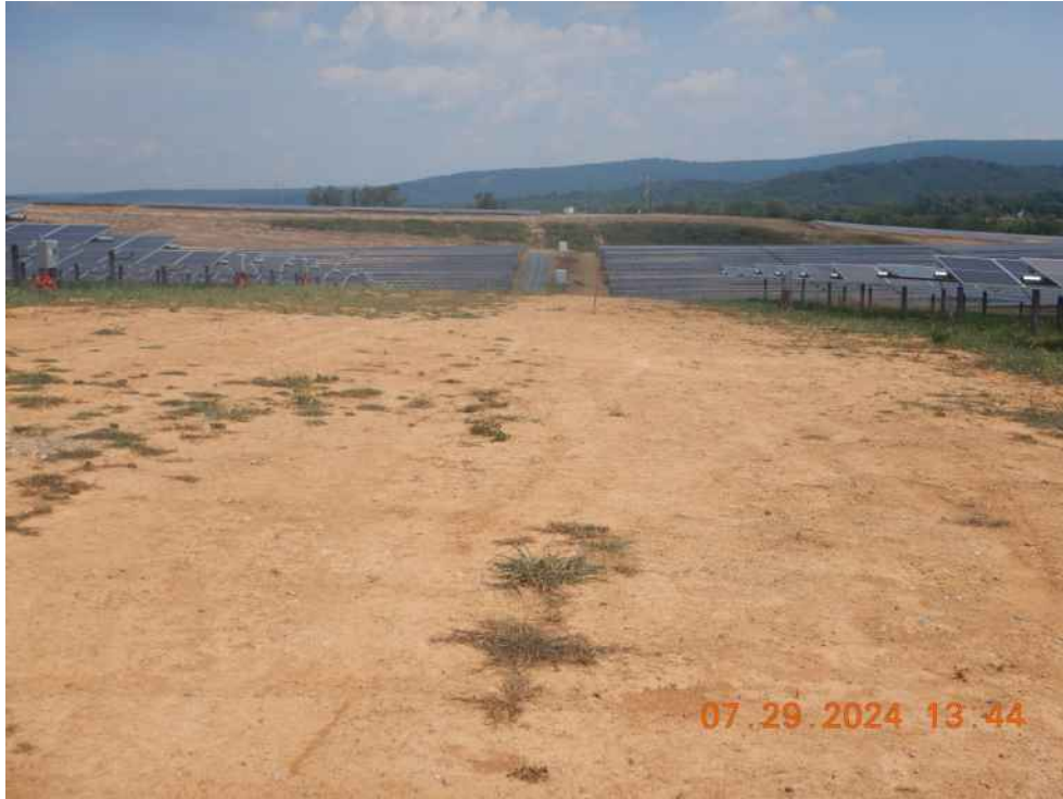
An unstabilized area that has not been actively worked. Sediment basin 13 drainage area.
