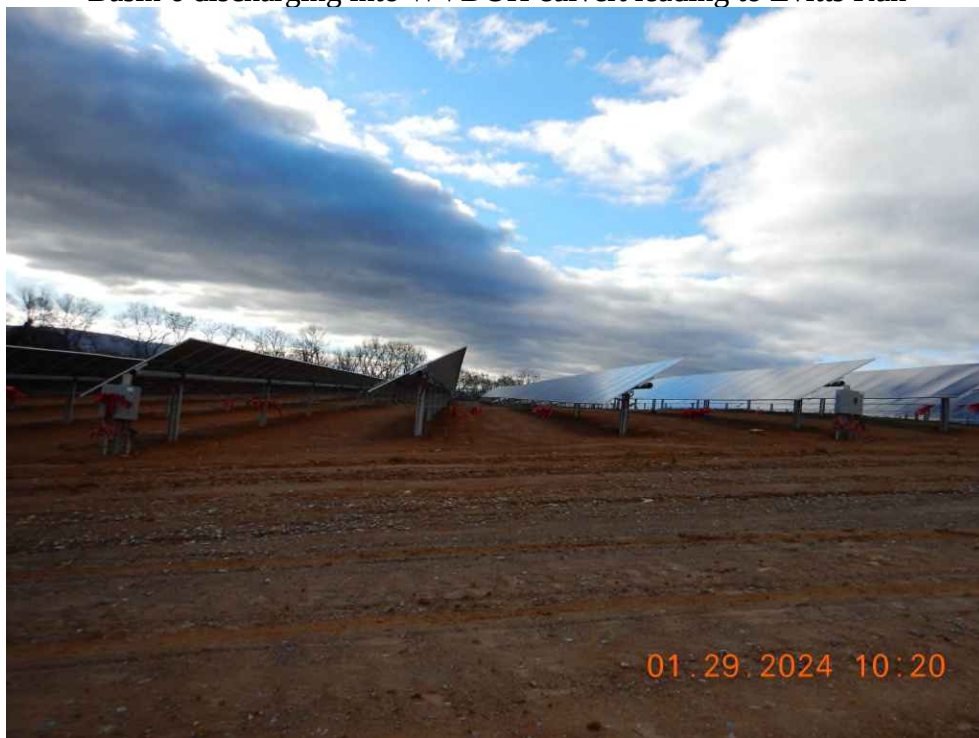
Area that has not been worked in the past 14 days and lacks stabilization.
