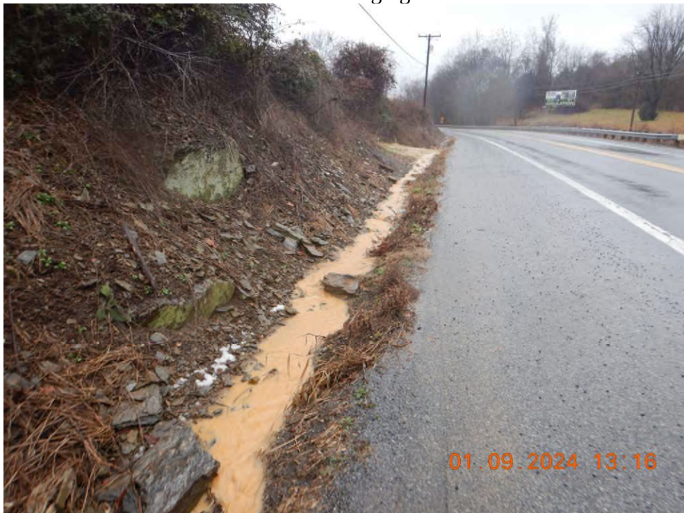
Sediment Basin 6 Discharging into WVDOH ditchline and discharging into WVDOH right of way leading to Shenandoah River.
