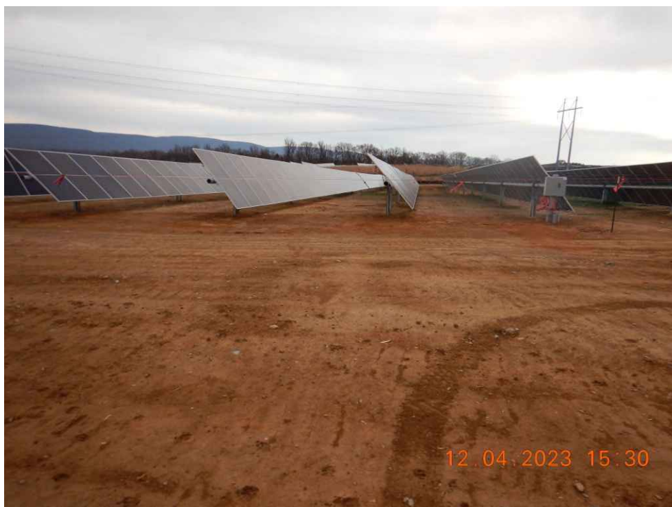
Area that has not been worked within the past 14 days and has not been stabilized.
