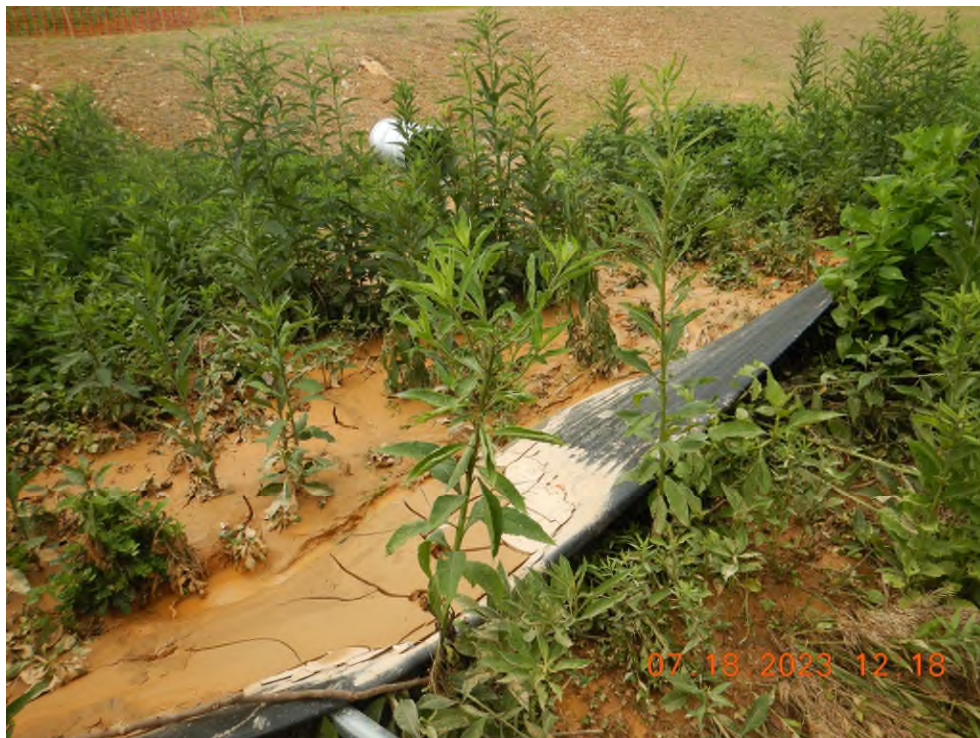
Super Silt fencing at lower end of outlet of Sediment Basin 6 needs maintenance
