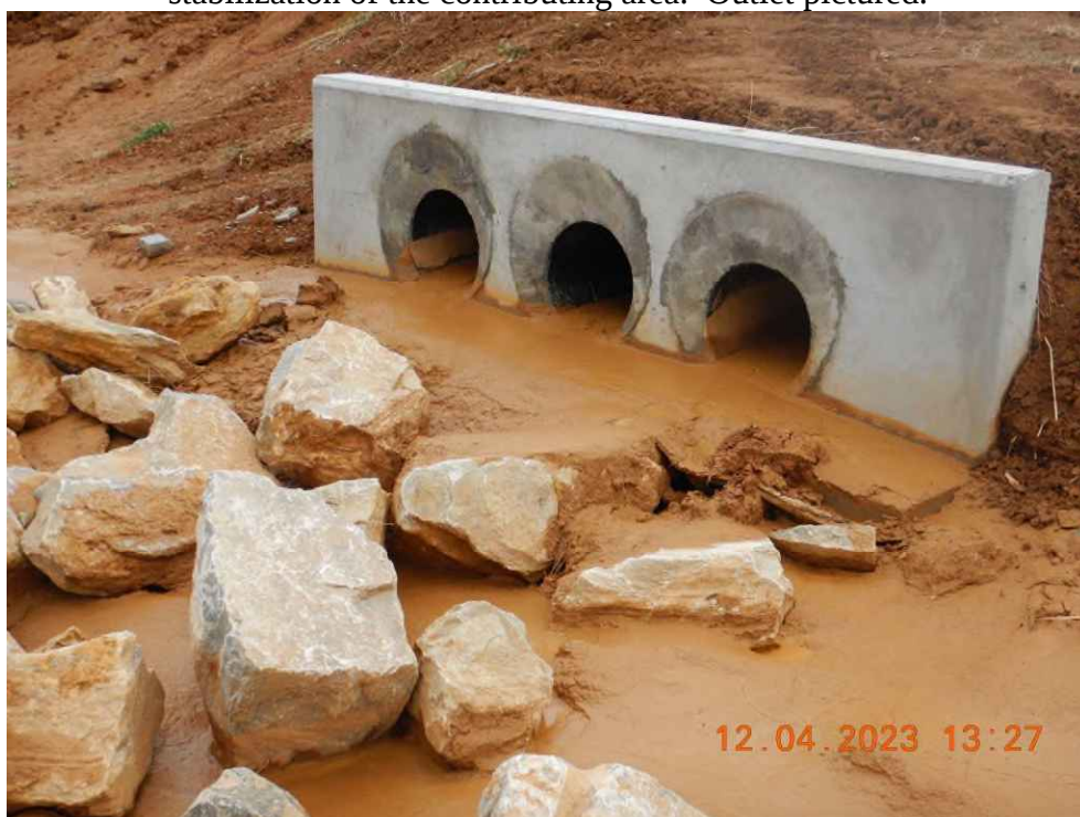
Sediment basin SB-11 (Pond 2B redline) that has been converted to stormwater retention prior to stabilization of the contributing area. Outlet showing sediment laden discharge pictured.
