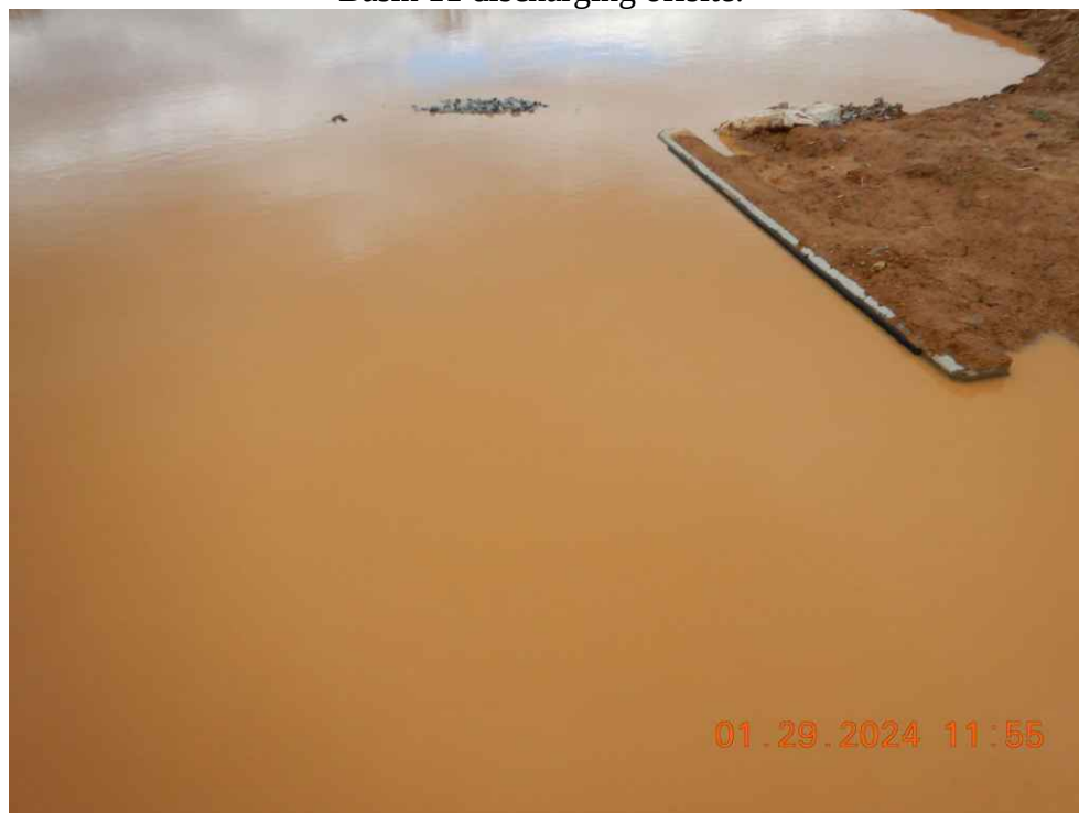
Basin 11 converted to stormwater management.
