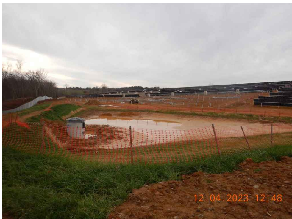
Sediment Basin 3 has been converted to Pond 3B prior to all upstream disturbance being vegetated.
