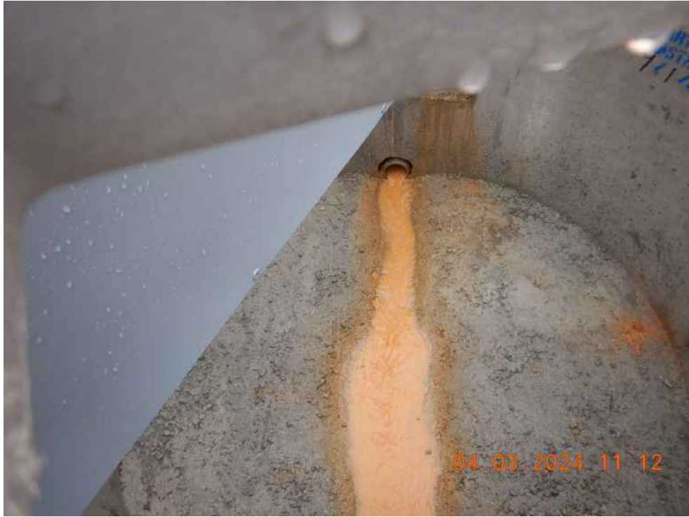
Structure for Pond 16A discharging sediment laden water.
