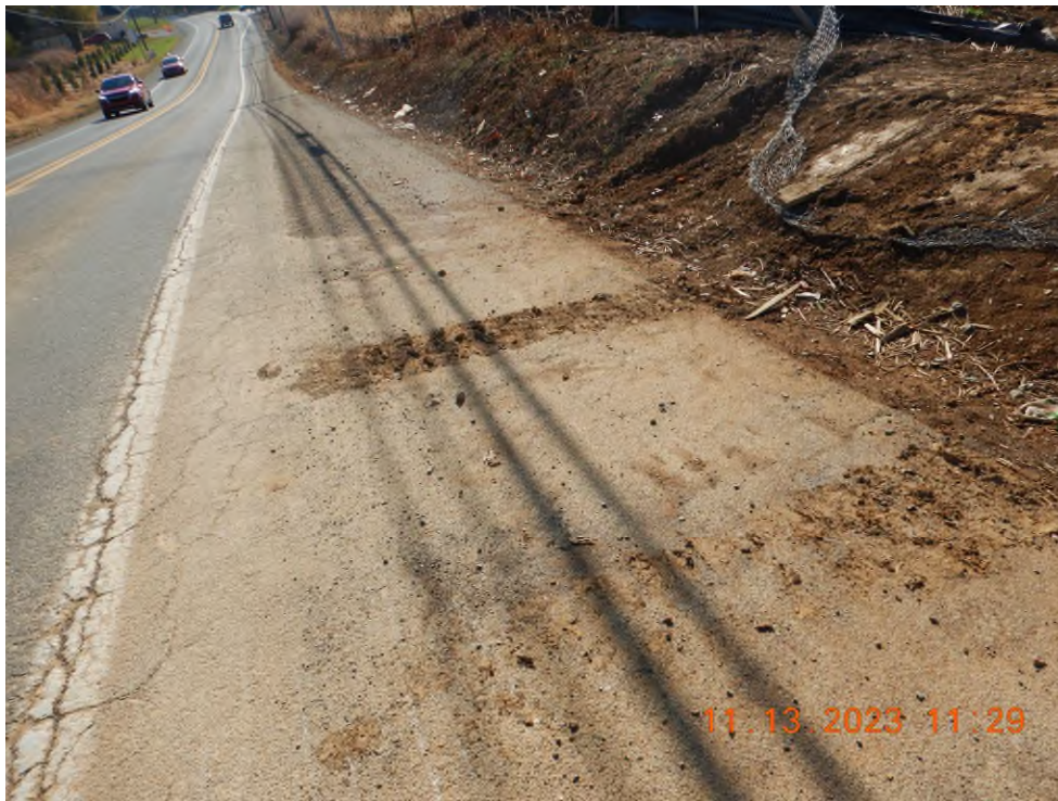
Track-out due to construction entrance not being stabilized.
