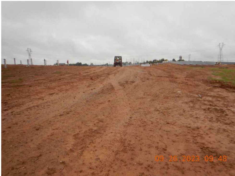
Unstabilized area of project. Temporary or permanent stabilization has not been started.
