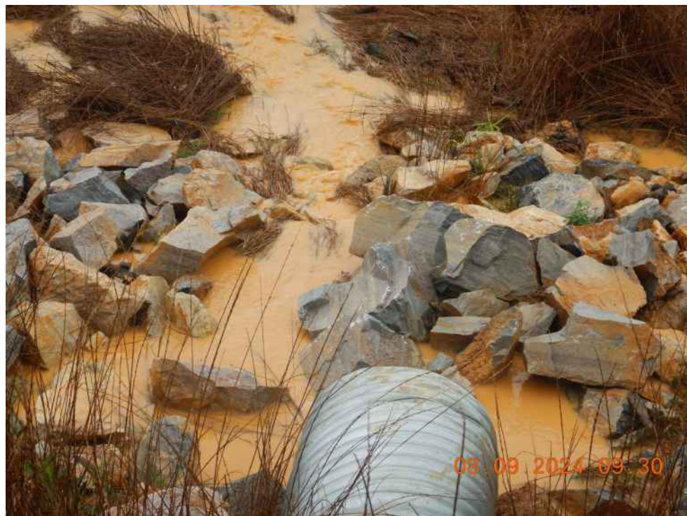
Sediment basin 12 discharging sediment-laden water into Evitts Run.
