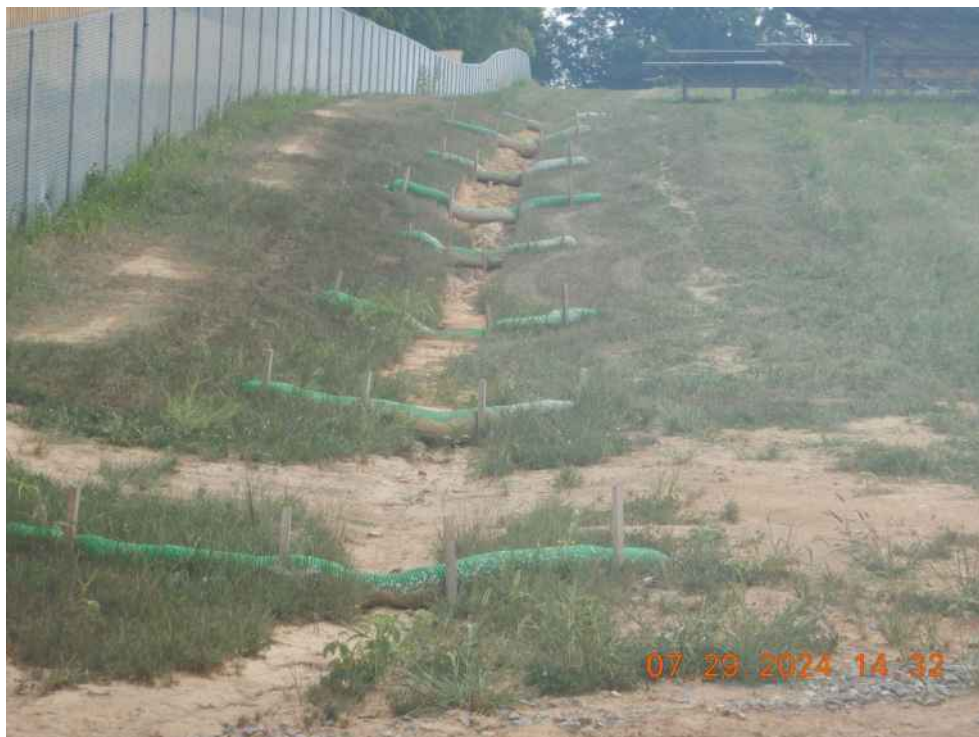
Diversion ditch checks that have been undermined and not repaired. Area of former access road below sediment basin 7.
