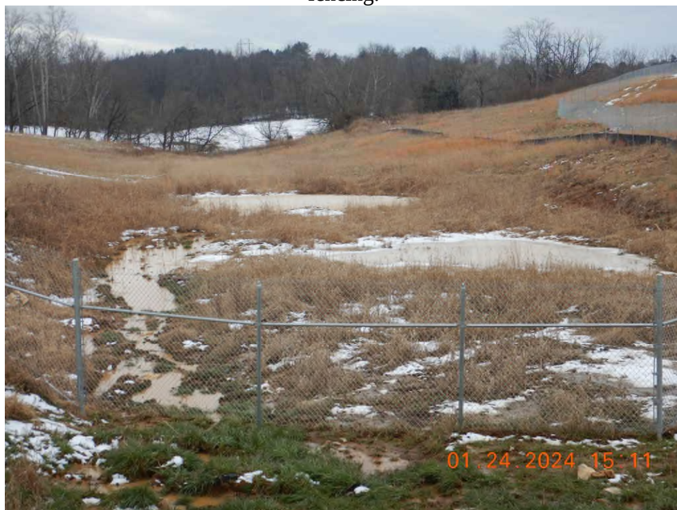
Sediment laden discharge into wetlands from Basin 13. Leading to Evitts Run.
