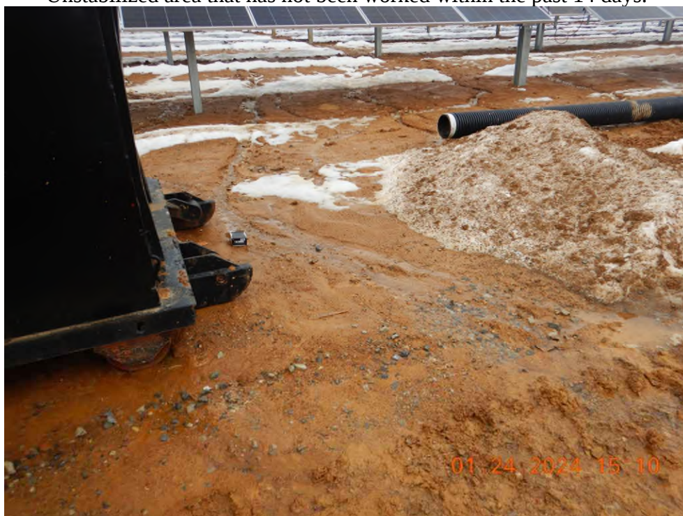
Erosion Rills that have formed above Basin 13. Area above has not been worked within the past 14 days.
