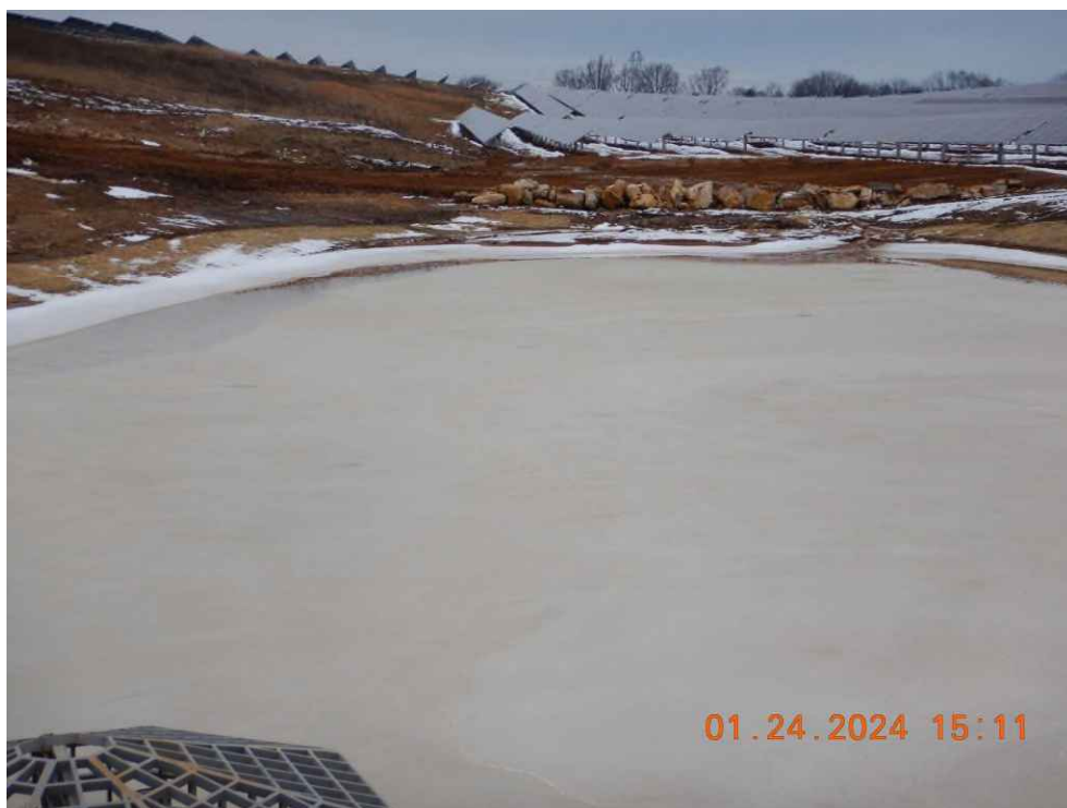
Area above Basin 13 is unstabilized prior to installation of the final stormwater feature.
