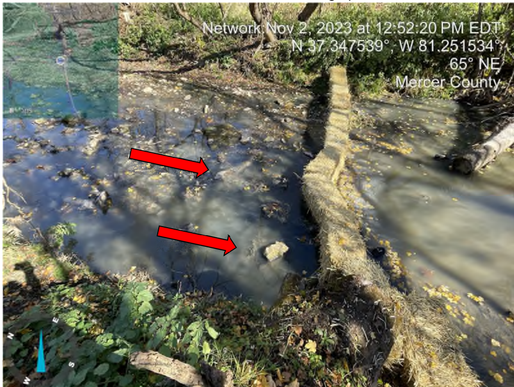
Failing containment of solids.
