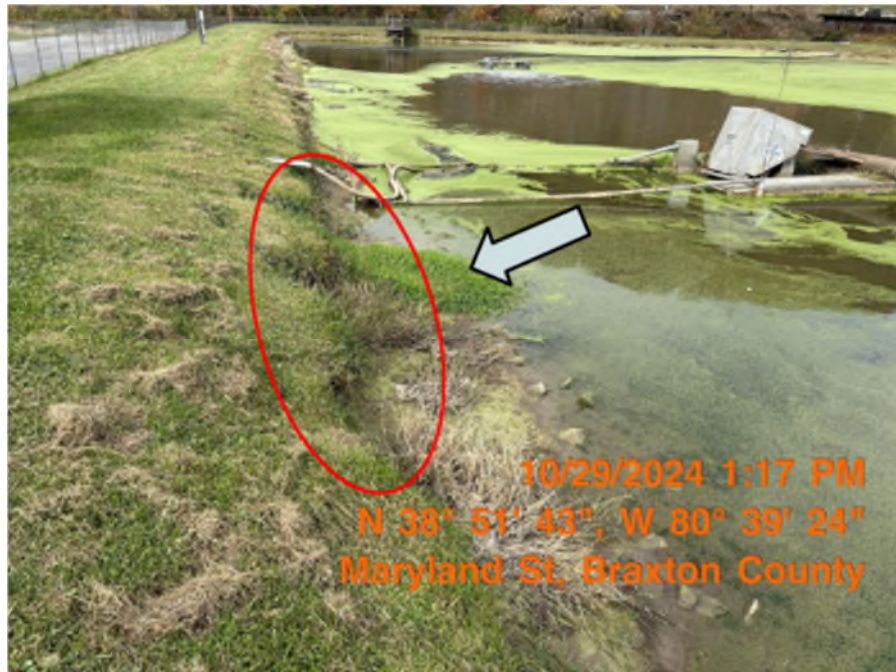
10/29/2024 – One of multiple areas where the dike was sloughing off into the lagoon.
