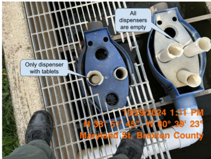
10/29/2024 – Empty chlorine tablet dispensers.
