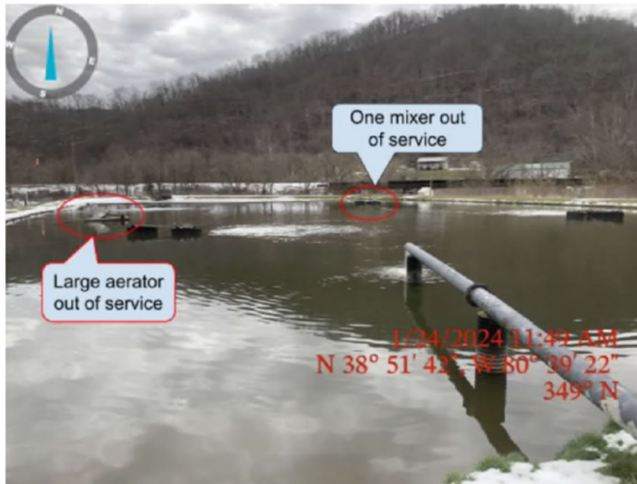
1/24/2024 – One mixer out of service and large aerator out of service.
