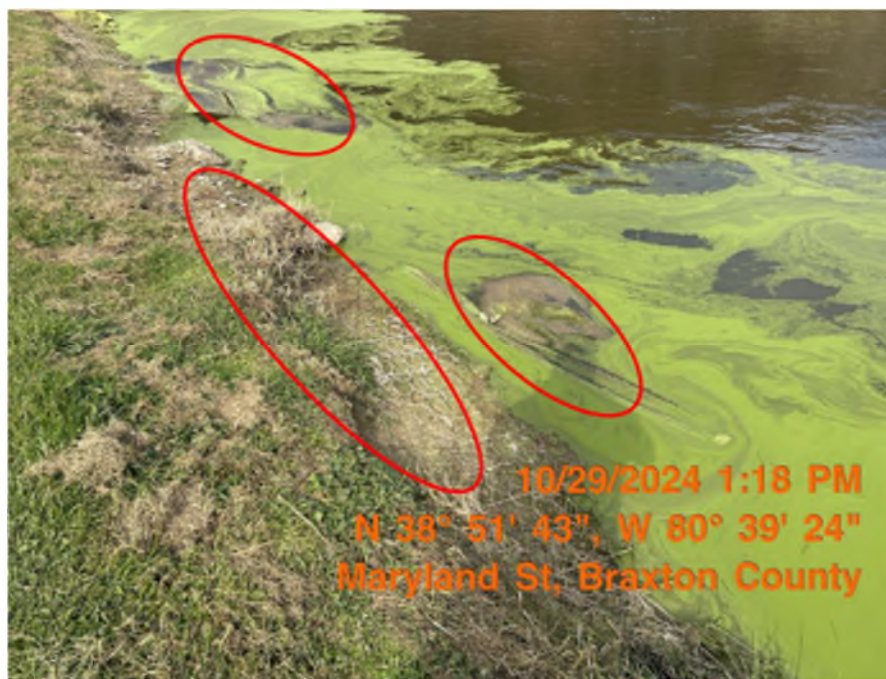
10/29/2024 – Metal framing exposed where liner pulled away. Bunched liner visible in lagoon.
