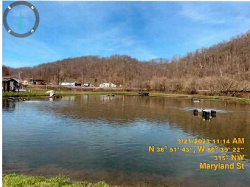
3/21/2023 – Large aerator was not functioning, and two mixers were in operation.
