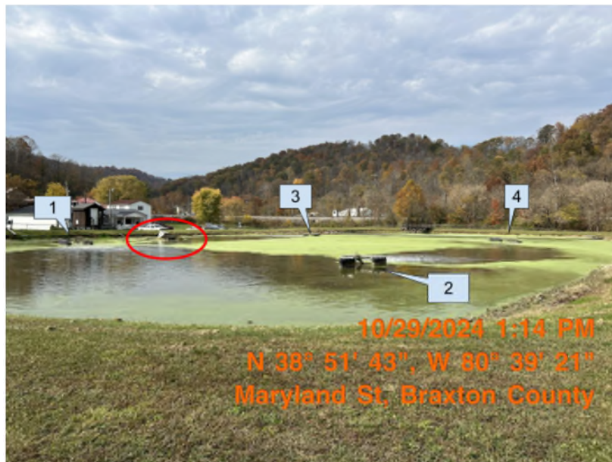
10/29/2024 – Mixer #4 was out of service, and the large aerator (circled) was not functioning.
