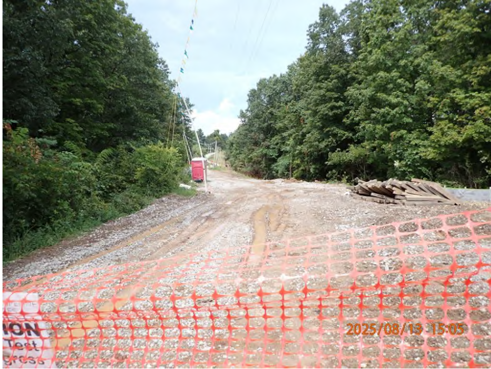
An access road that traverses to Station Marker 31+00 and TAR-3 and is not part of the approved SWPPP.
