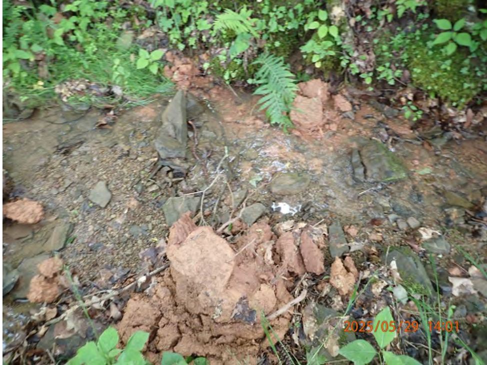
Sediment deposits in the UNT of Stackpole, causing Conditions Not Allowable (CNA) ( 39^{\circ} 28'07'' N, -80^{\circ} 41'49'' W), due to failure to install perimeter controls and outlet treatment between Station Markers 37+00 and 46+00.
