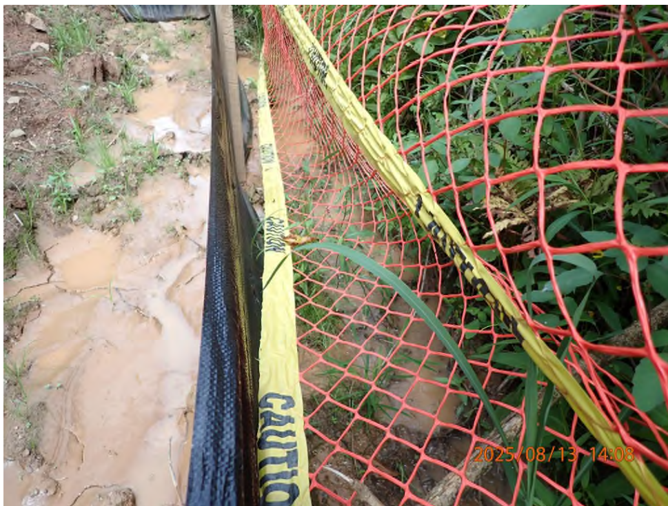
Sediment laden water discharged into the Wetland UNT of Lefthand Fork of Stackpole Run, causing CNA (39° 27'56" N, -80° 41'24" W).
