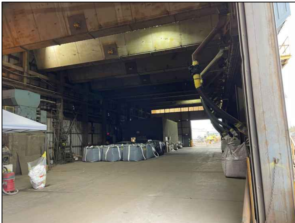
Photo #4 – November 18, 2024: Super sacks of K061 hazardous waste and filling area in east baghouse.
