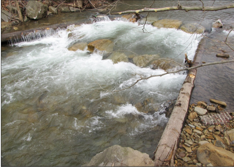
This structure on pre-law mining-impacted Buffalo Creek in Logan County is helping restore the stream to the days when trout fishing was plentiful.
