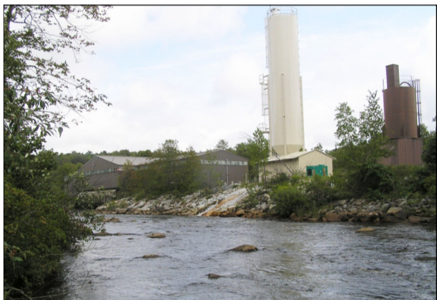
AML's newest doser on the Blackwater River is flanked by the original limestone drum station (left) and an outdated doser.
