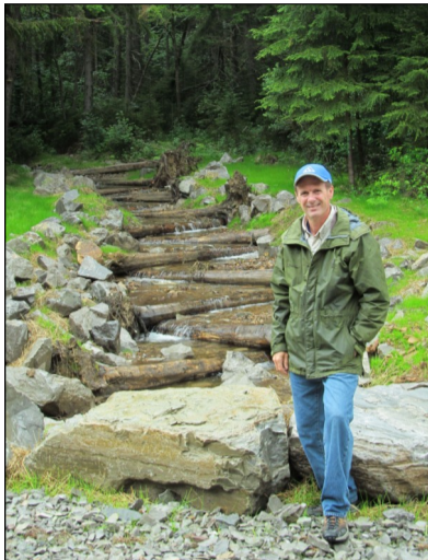
The DEP’s Ed Hamrick stands near a natural stream restoration step-pool complex entering the baffled fish passage culvert on Lamothe Run.
