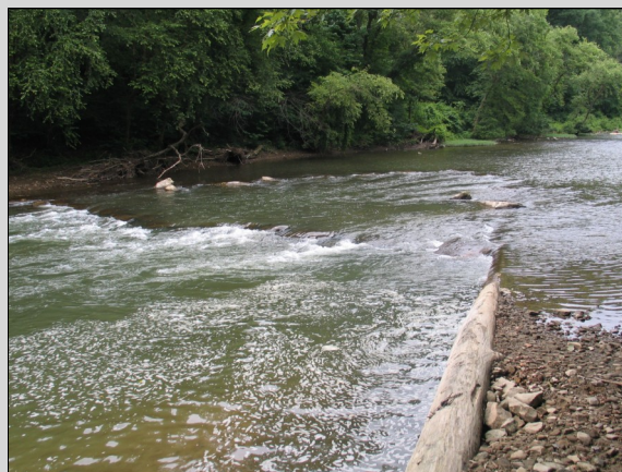
The cross vane design of the restoration structures on the Little Coal narrows the river and speeds up current.
