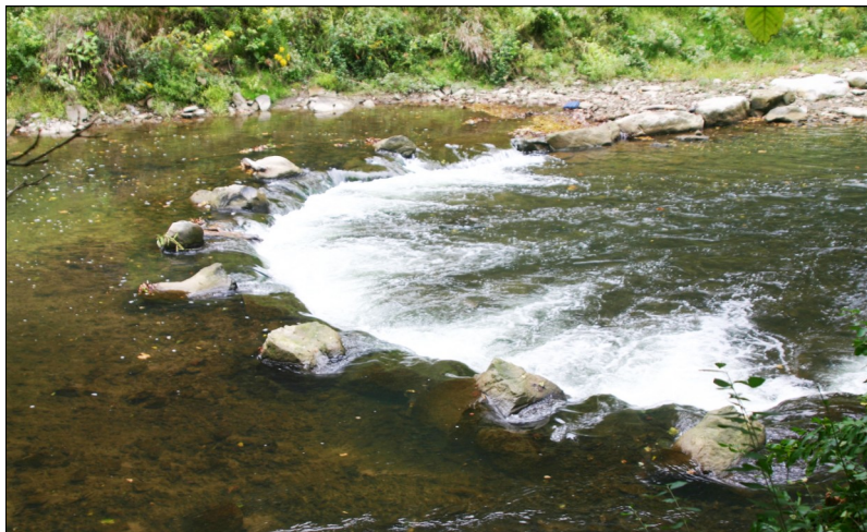
The Little Coal River project will include restoration structures similar to this, which are already in place on several miles of the river. The structures are designed to speed up the current on the Little Coal and improve habitat.
