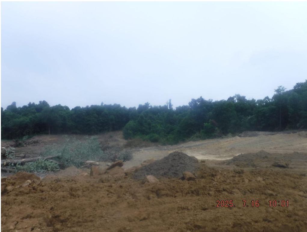
Photo # DSCF5391: Site overview
