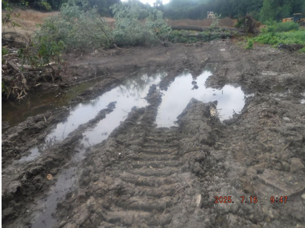
Photo # DSCF5386: Sediment deposits in UNT Mahan Run at or near N 40° 20.5518', W 80° 35.7354'.
