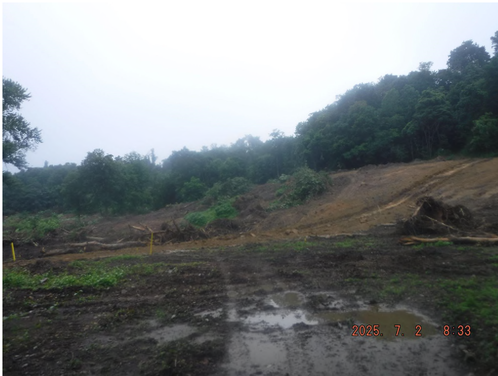
Photo # DSCF5063: Site overview
