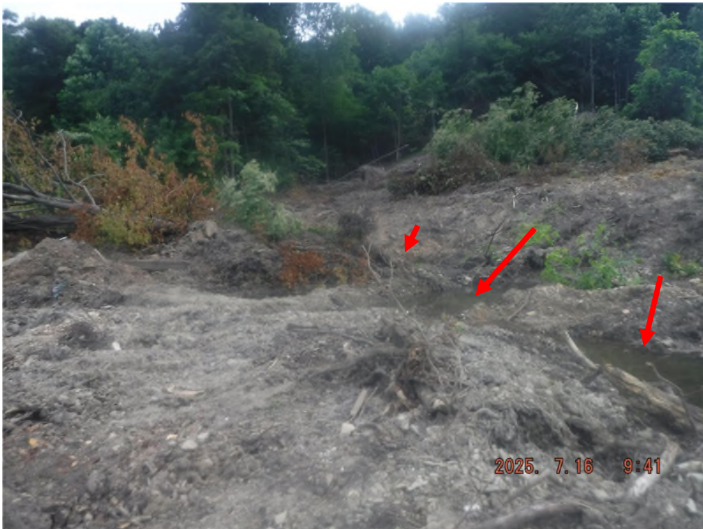
Photo # DSCF5367: Looking upstream of N 40° 20.5848', W 80° 35.7501' along UNT Mahan Run (stream labeled by arrows) with sediment deposits and no E&S controls.
