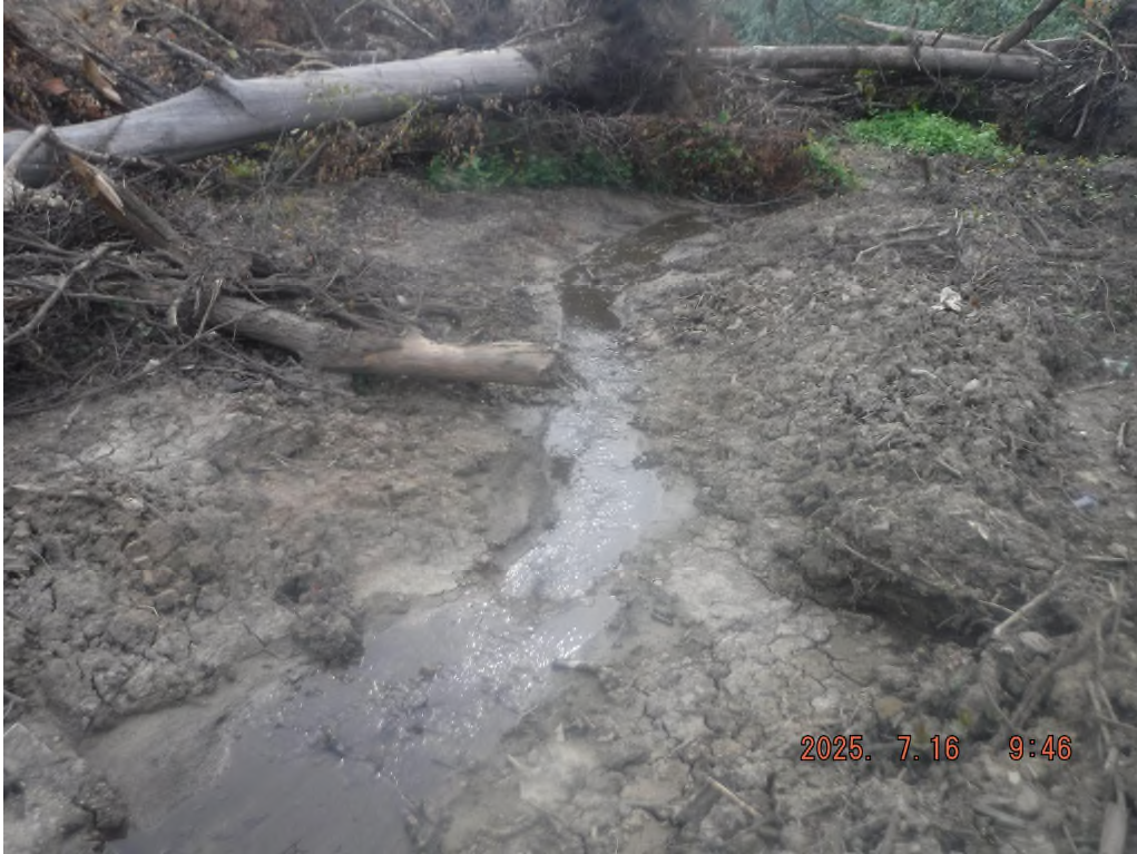
Photo # DSCF5380: Sediment deposits in UNT Mahan Run at or near N 40° 20.5686', W 80° 35.7457'
