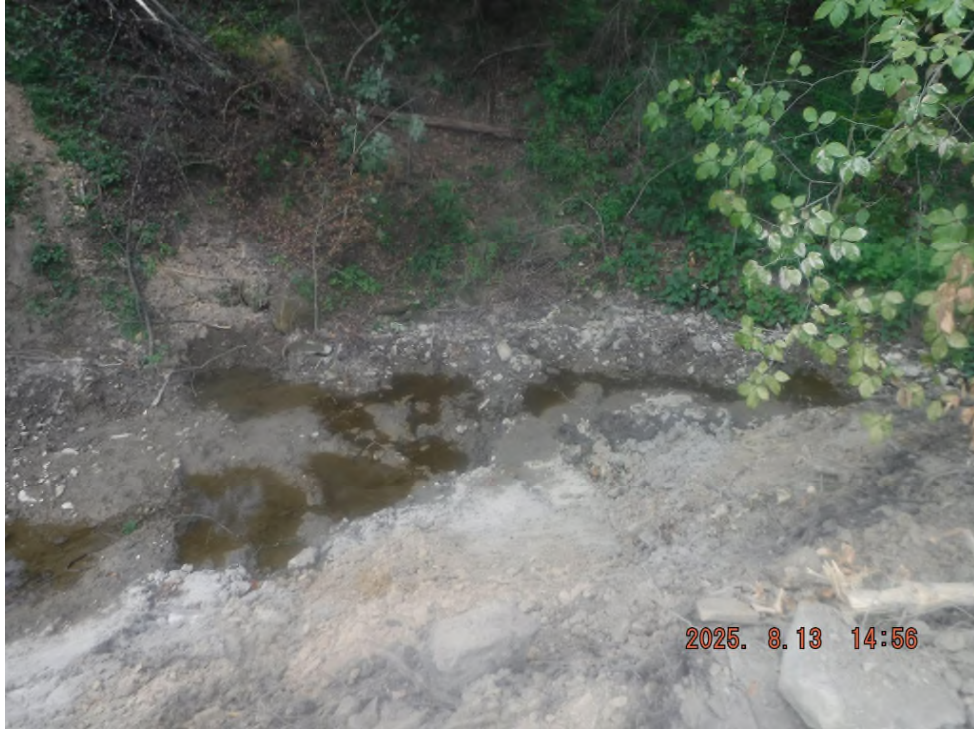
Photo # DSCF6180: Sediment deposits in UNT Mahan Run at or near N40° 20.6255', W80° 35.7453'
