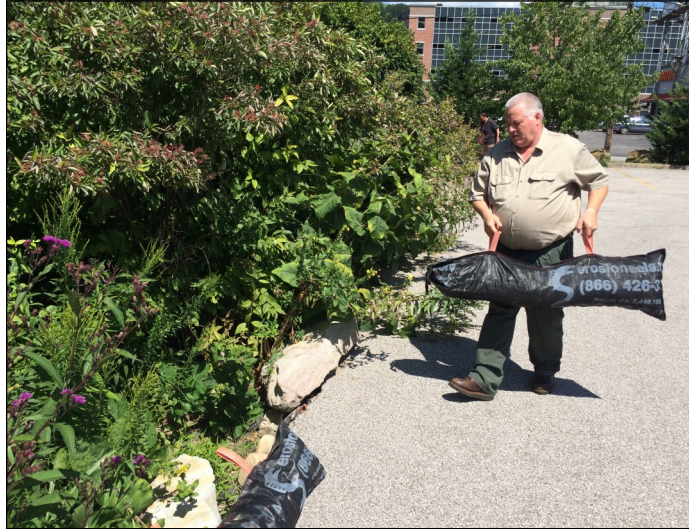
Larry Board, an environmental resources specialist with the Division of Water and Waste Management, places a new erosion eel beside the DEP’s rain garden to help keep pollutants out.
